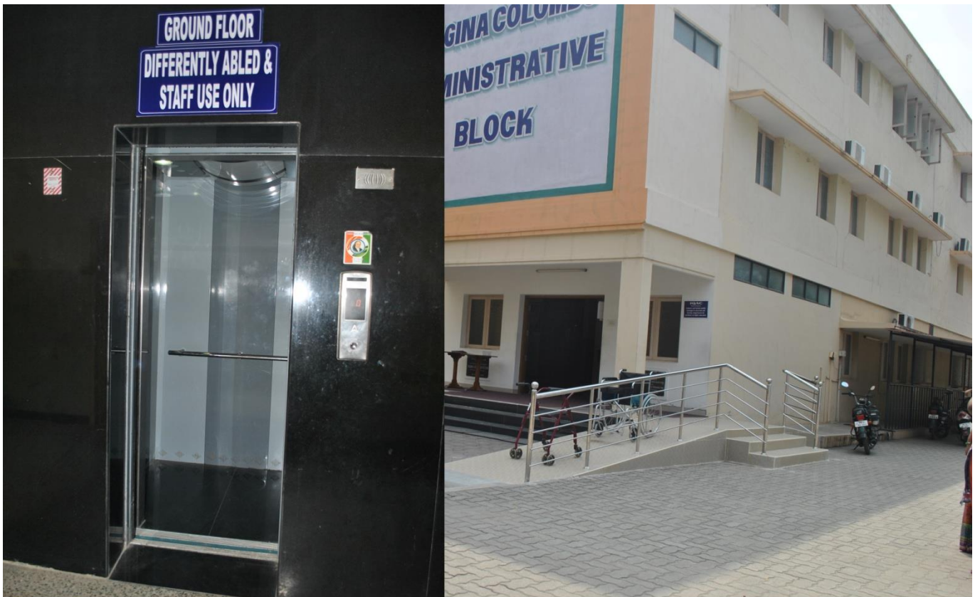
Elevator and Ramp facilities available at the Admin Block
