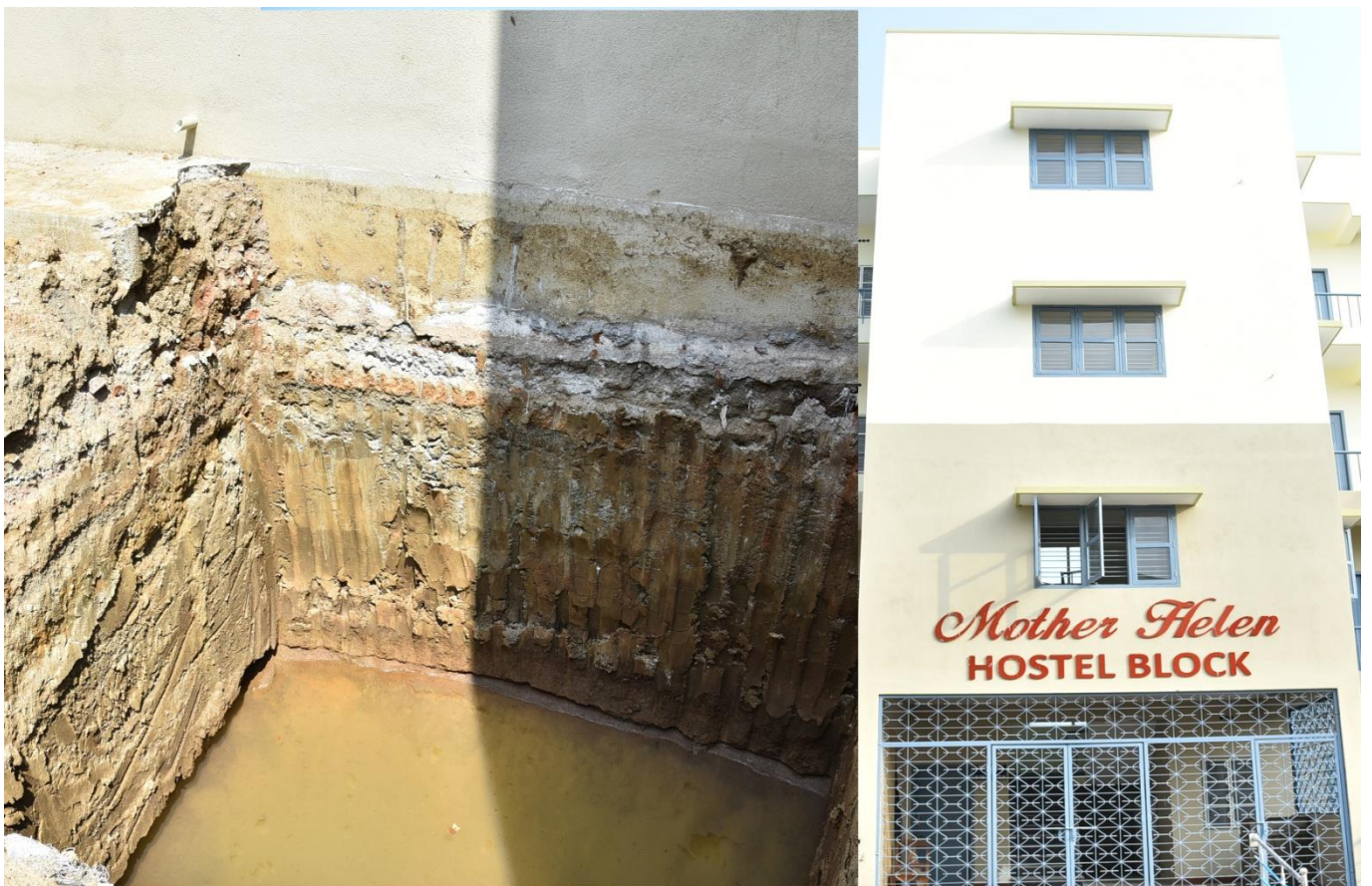
Elevator under construction in the Hostel Block
