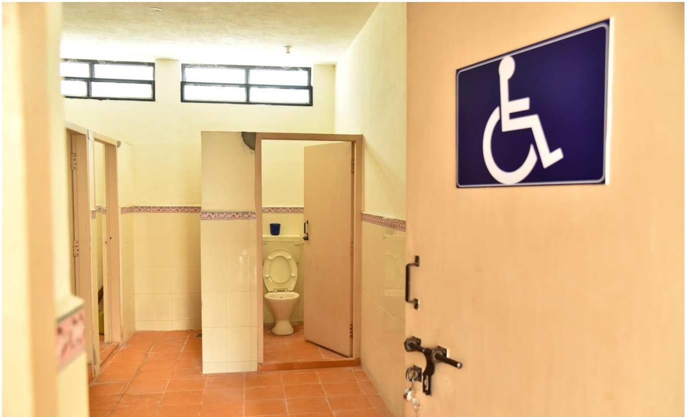
Special Lavatory facility available at the First Floor in Admin Block
