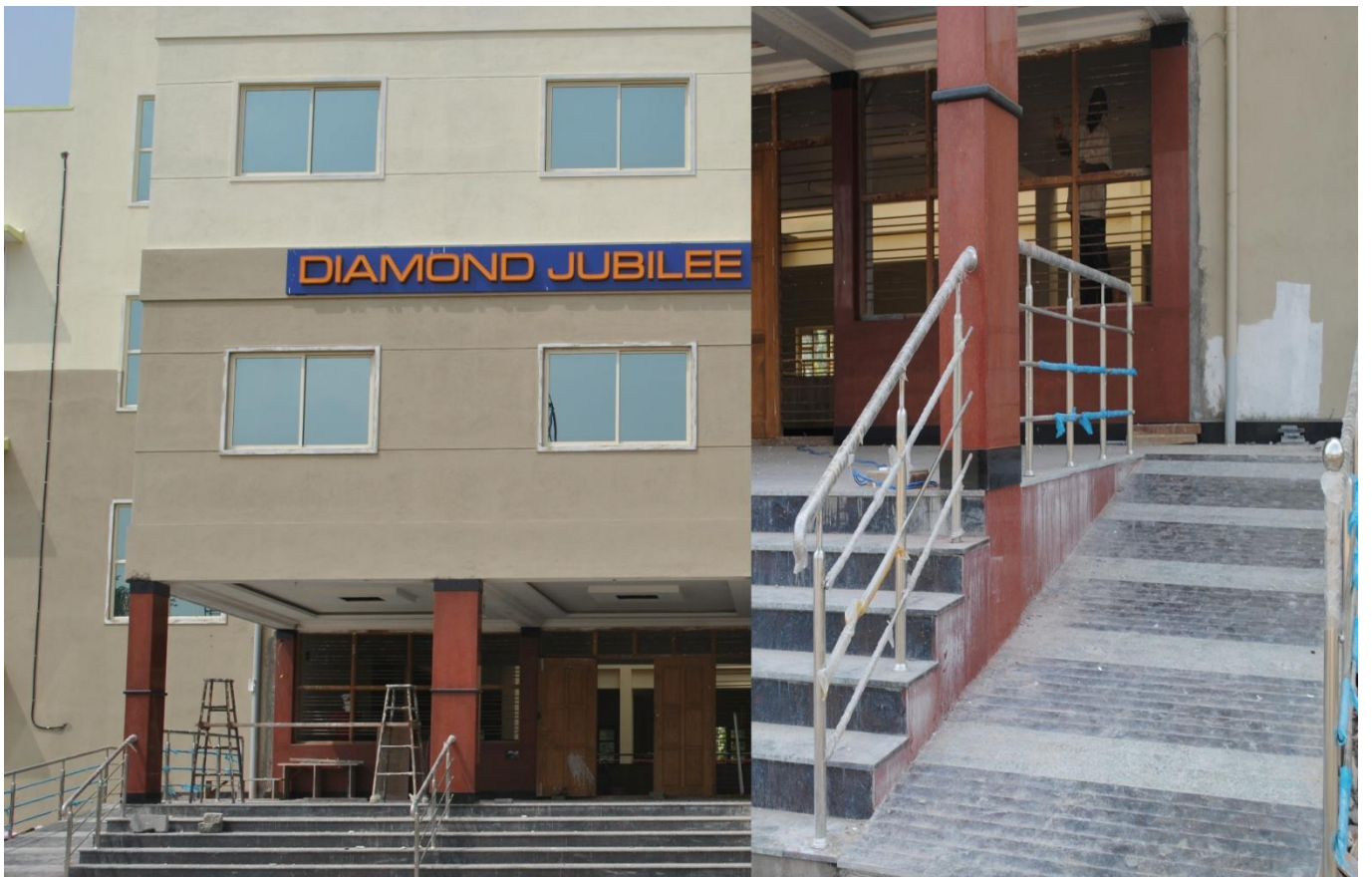
Elevator and Ramp facilities available in the Library Block
