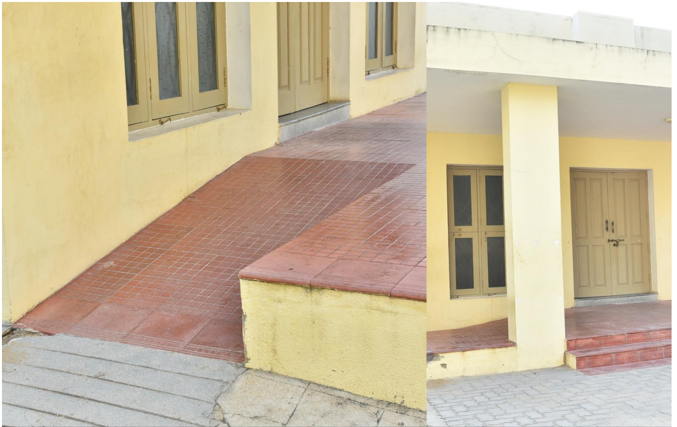
Ramp facility available at the College Canteen
