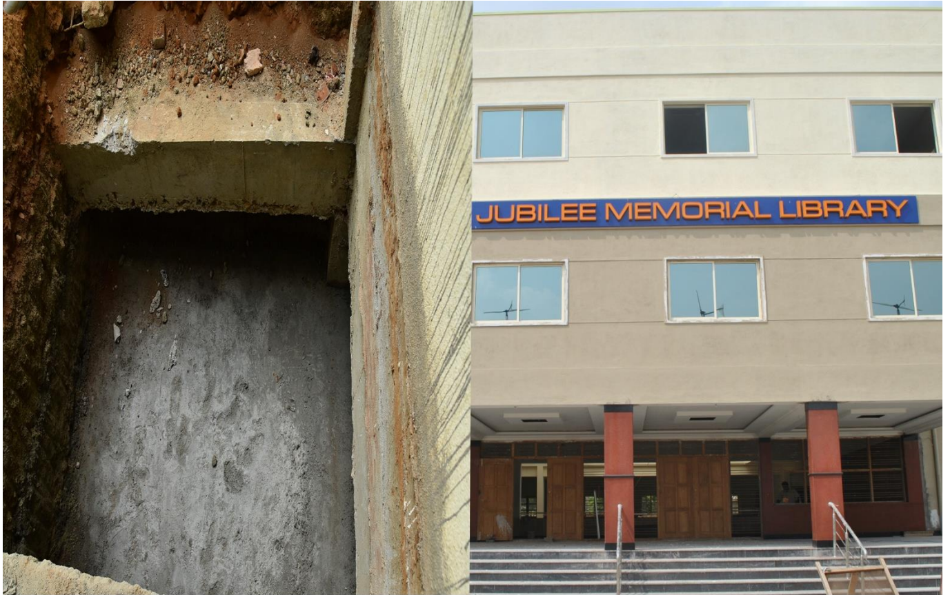
Elevator under construction in the Library Block
