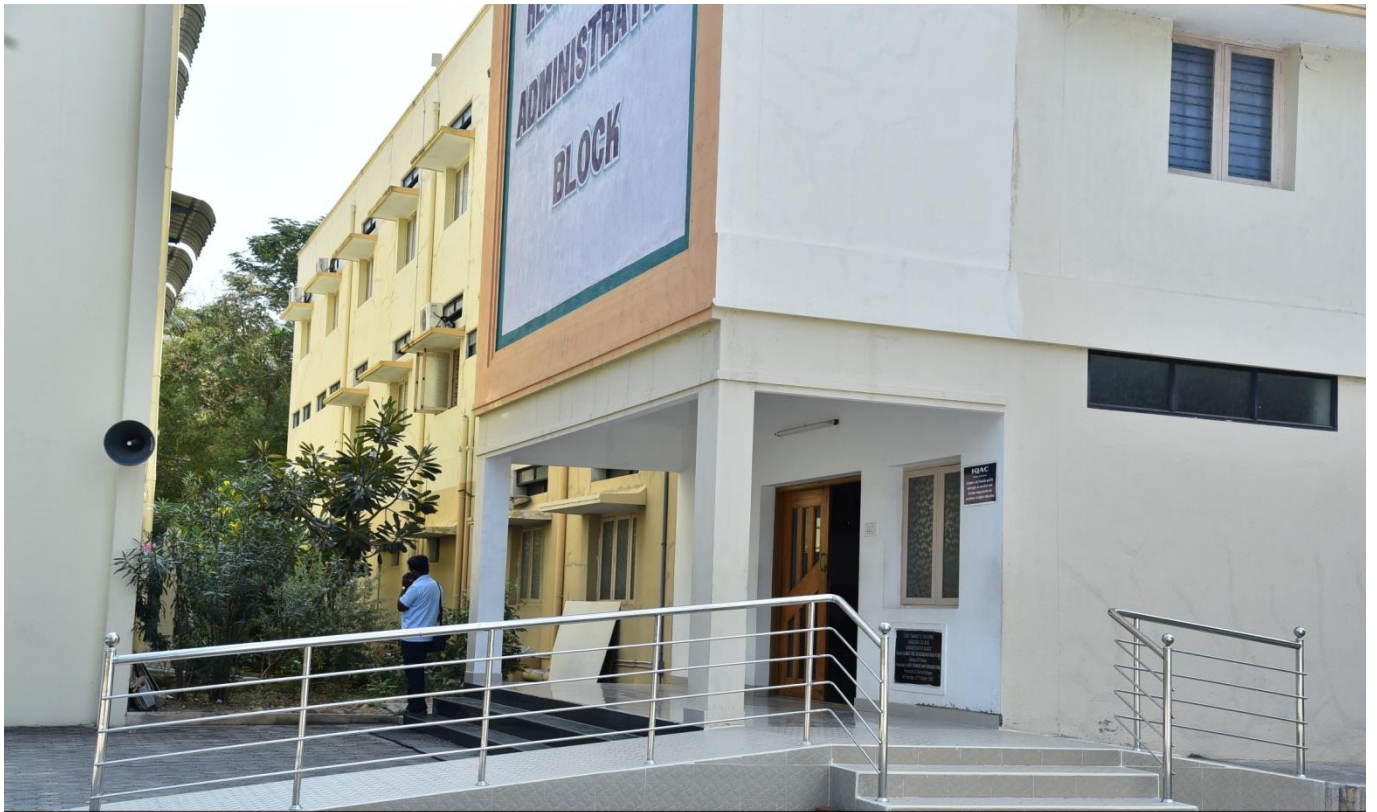
Regina Colombo Administrative Block Elevator and Ramp facilities
