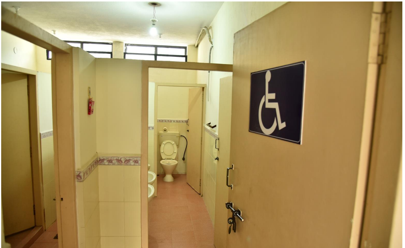
Special Lavatory facilities available at Ground Floor Admin Block
