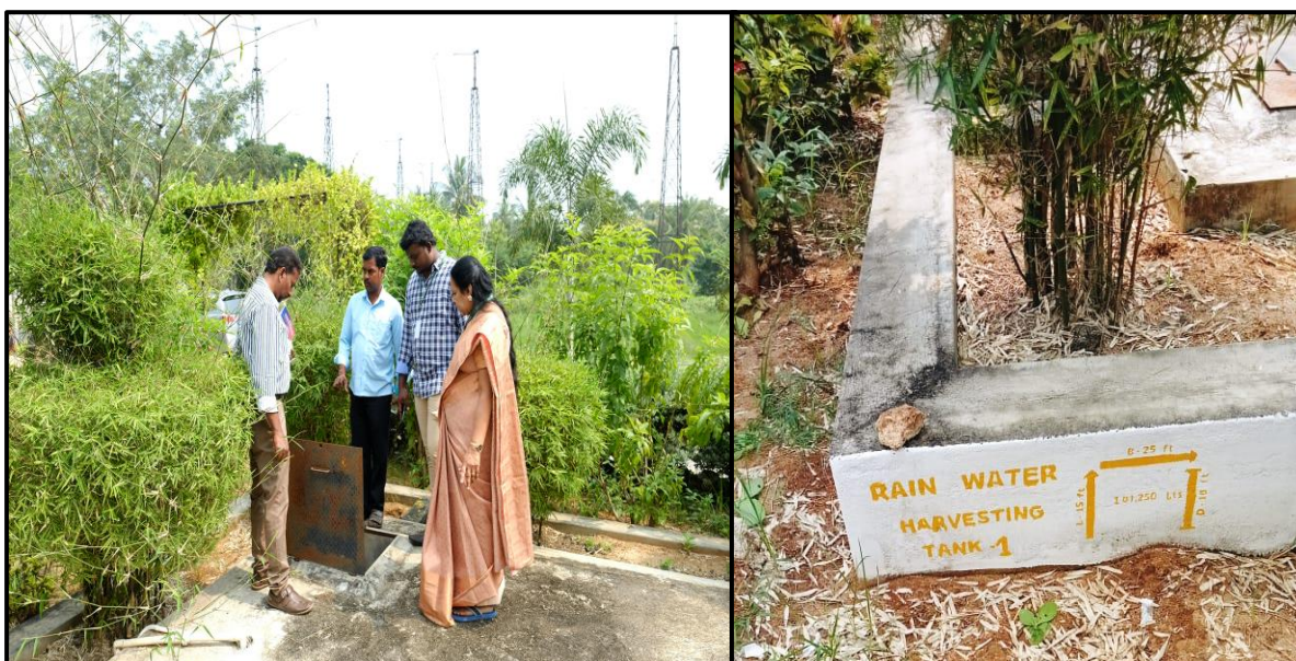
Rainwater Harvesting units in Auxilium College (Autonomous), Vellore - 632 006, Tamil Nadu.
